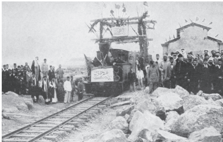
Extending the imperial reach. Opening of Hijaz Railway.
